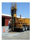
dated drilling. Air rotary capability can be added to our auger rigs to advance the bore hole beyond normal refusal conditions. Projects that require borings over water surfaces can be completed using a variety of barge mounted units.
